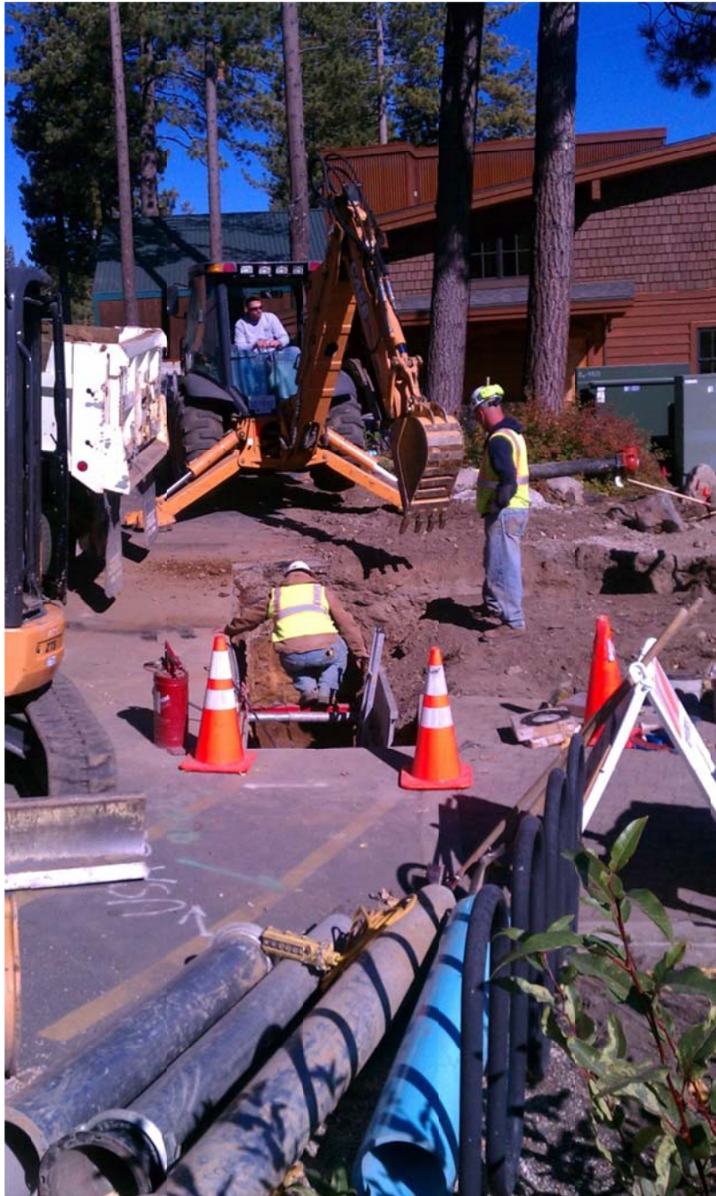
Fire Hydrant Install
