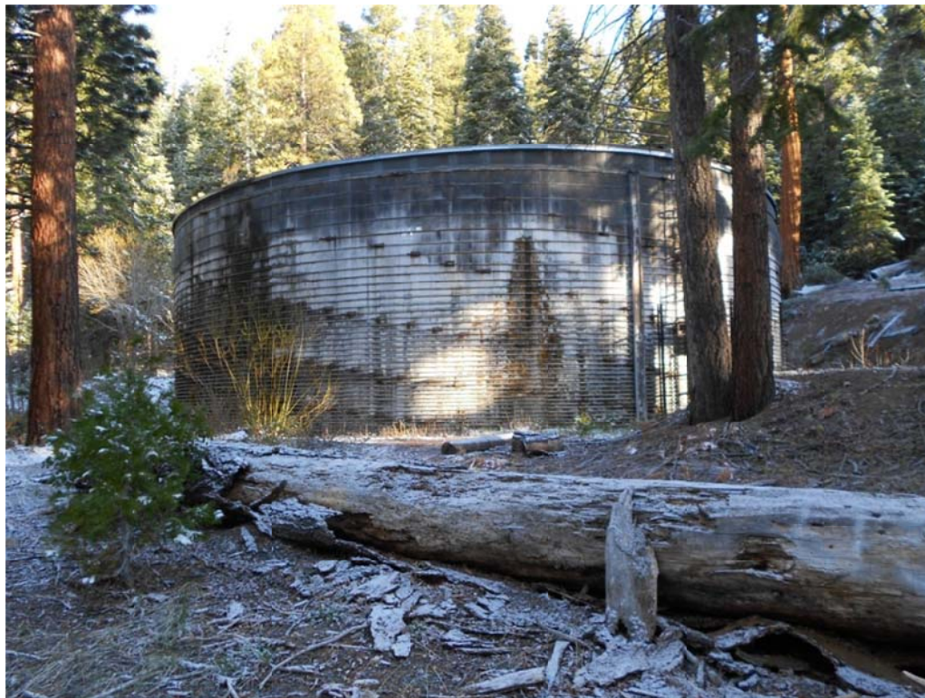
Bunker Water Tank - Capital Project No. 8151
